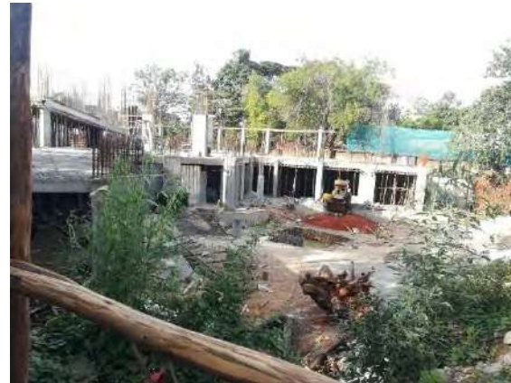
Column rebar work on ground floor underway.
