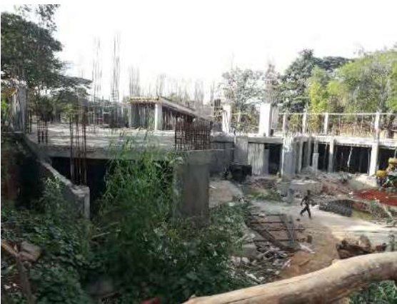
Formwork on sections of ground floor underway.
