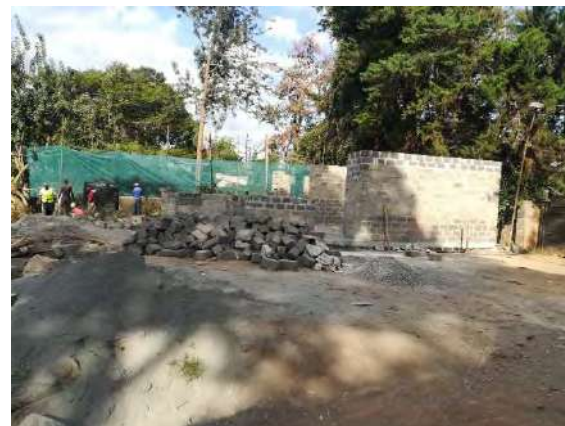
Blockwork on show house unit underway.
