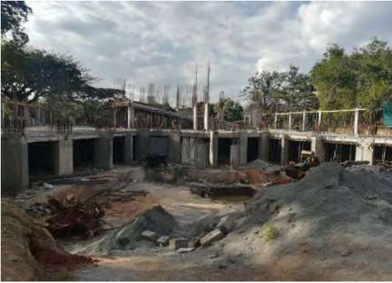
Slab casting on sections of basement done.
