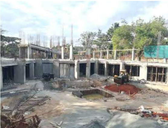
Beam reinforcement work on parts of ground floor underway.
