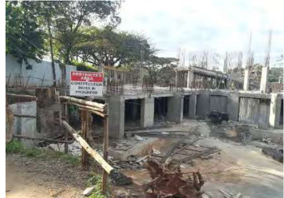
Structural elevation work for ground floor underway.
