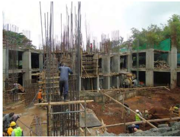
-View of ground & basement floors.
