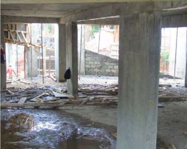
Interior View of basement.
