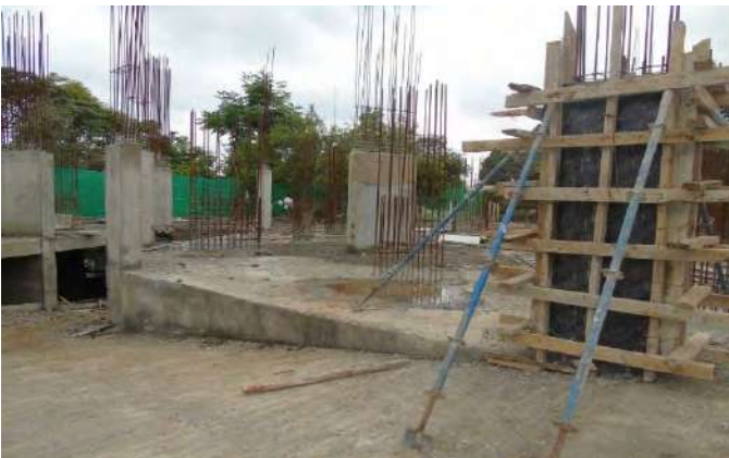
-Elevation work for 1 st floor underway.
