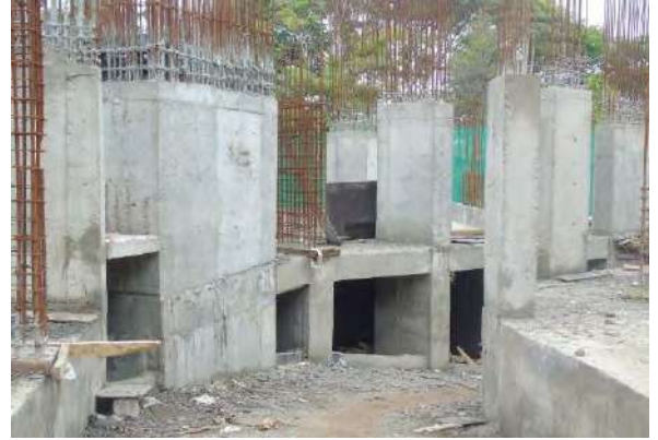
-Column rebar work on ground floor shutter underway.
