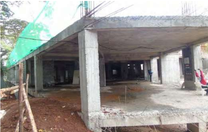
-Interior view of ground floor, shuttering work done.
