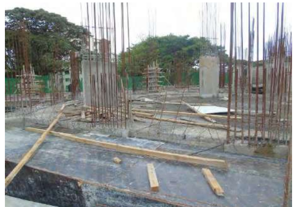
-Formwork for shuttering parts of ground floor underway.
