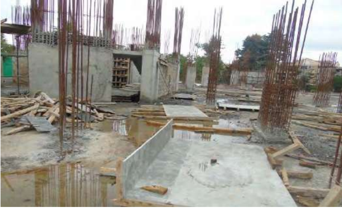
-Structural elevation work for elevation of 1 st floor underway.
