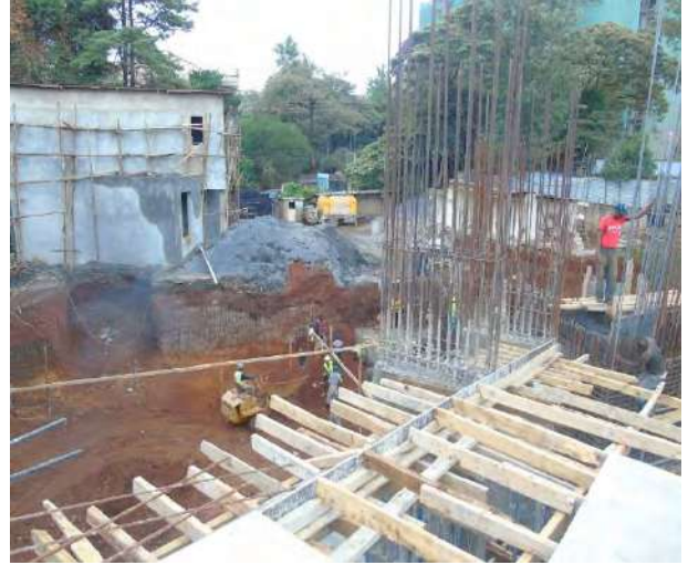
-Ground excavation for elevation of parts of basement floor underway.
