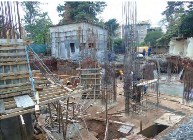
-Structural elevation work on parts of basement floor underway.
