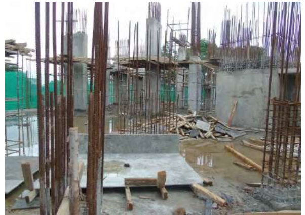
-Beam & column rebar work for elevation of 1 st floor underway.
