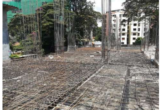
-Slab casting on parts of 1 st floor underway. (Ground floor shutter).
