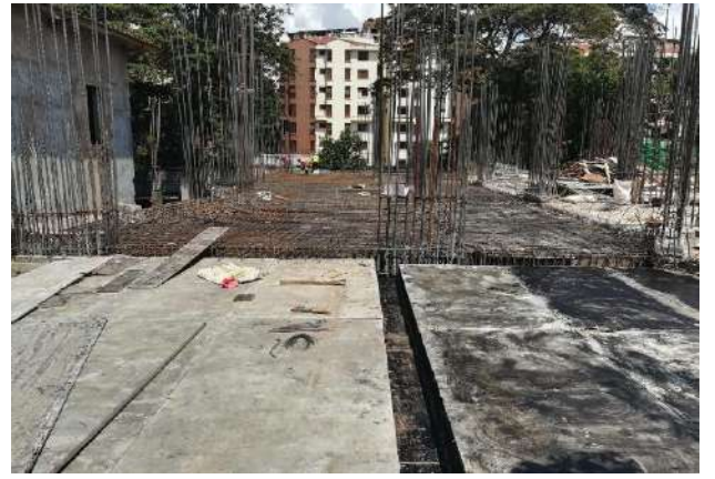
-Column & beam rebar work underway.
