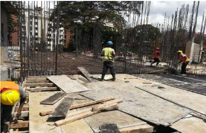
-Formwork for slab casting on parts of 1 st floor underway.
