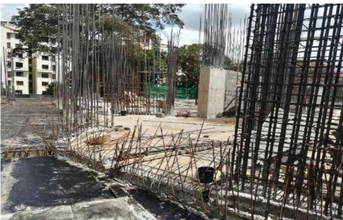
-Column & beam concreting work underway.
