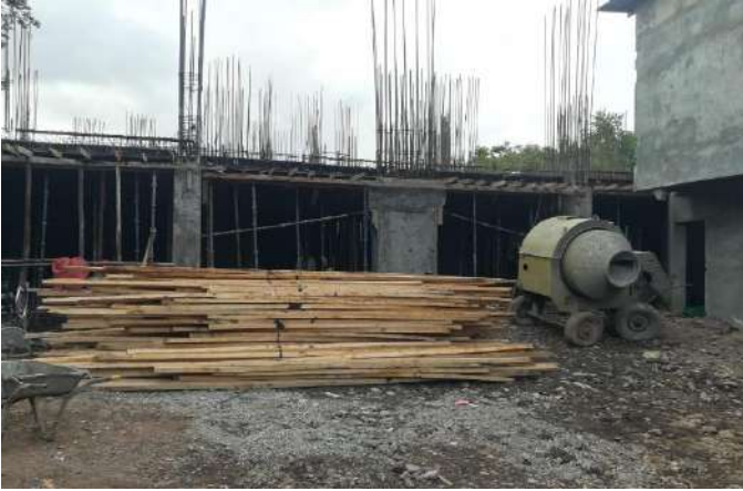
-Column rebar work on parts of 1st floor underway.(Ground floor shutter).
