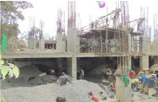
-Column casting for 2 nd podium floor done.
