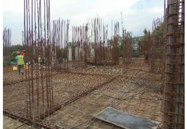
-Column & beam rebar work on 2 nd podium floor underway.
