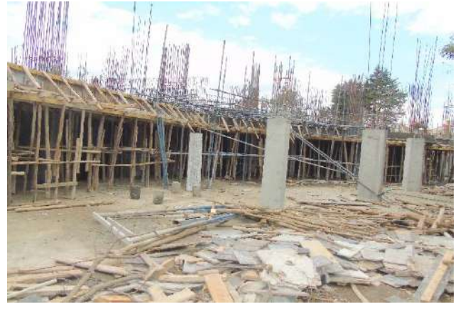
-Structural elevation work on 2 nd podium floor underway.
