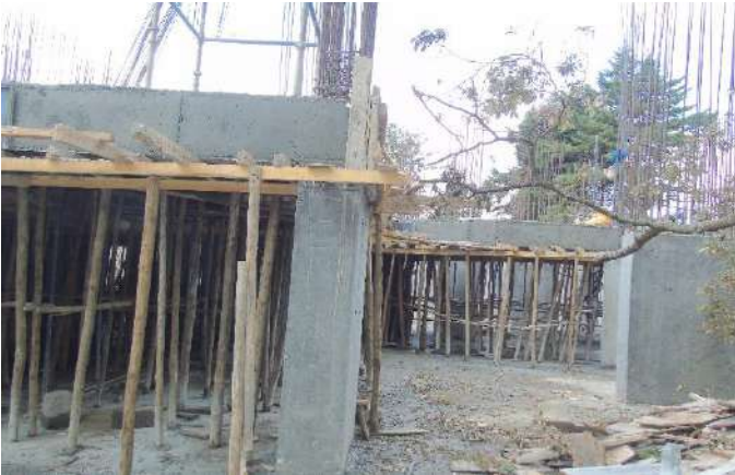
-Column casting for 2 nd podium floor done.
