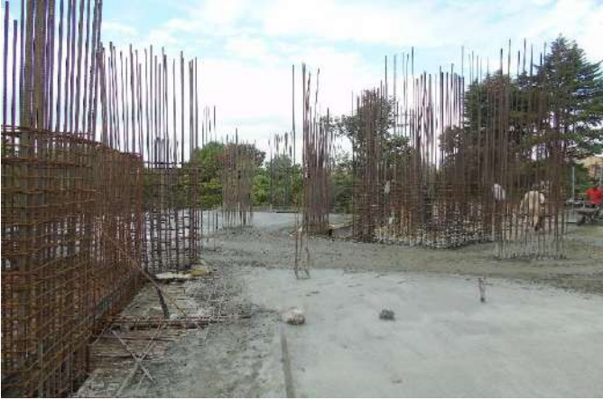
-Slab shuttering on parts on 2 nd podium floor underway.
