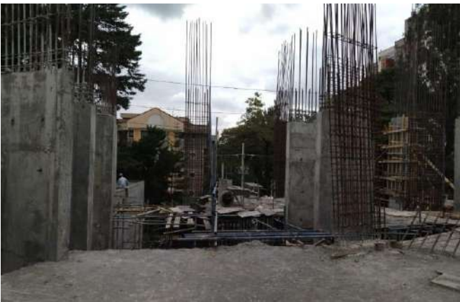
-Column casting for elevation of amenities floor done.
