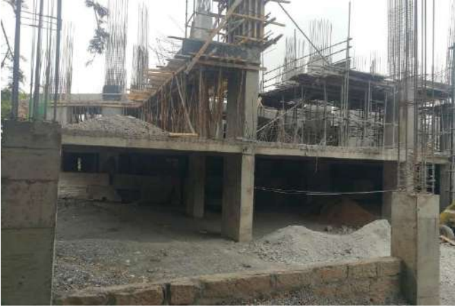
-Slab casting on parts of 2 nd floor (Amenities floor) underway.
