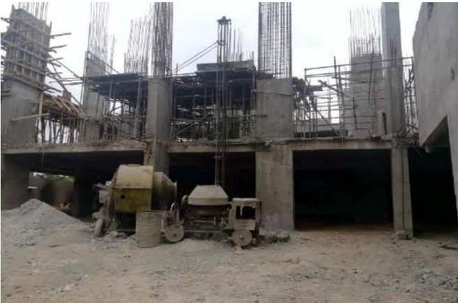
-Column casting for elevation of amenities floor done.
