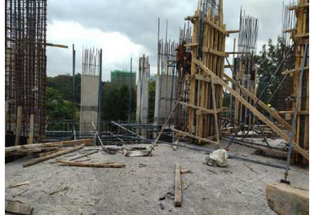
-Column & beam rebar work on 2 nd floor (Amenities floor) underway.
