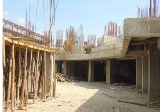
-Column & beam rebar work on 2 nd floor (Amenities floor) underway.
