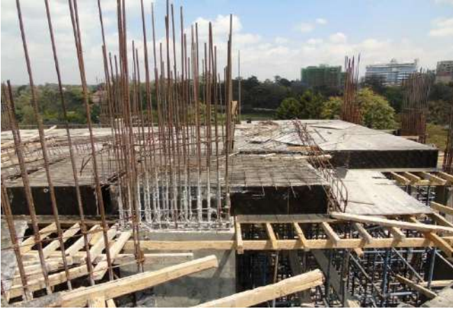
-Formwork for shuttering parts of 2 nd floor (Amenities floor underway.)
